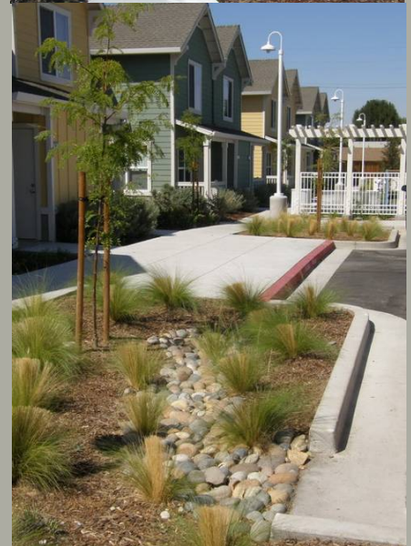
Natural stormwater filtration
