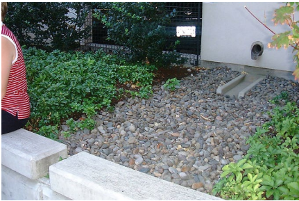
Roof drain routes to permeable landscaping
