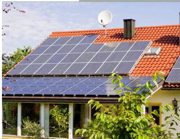
Solar panels as afterthought
