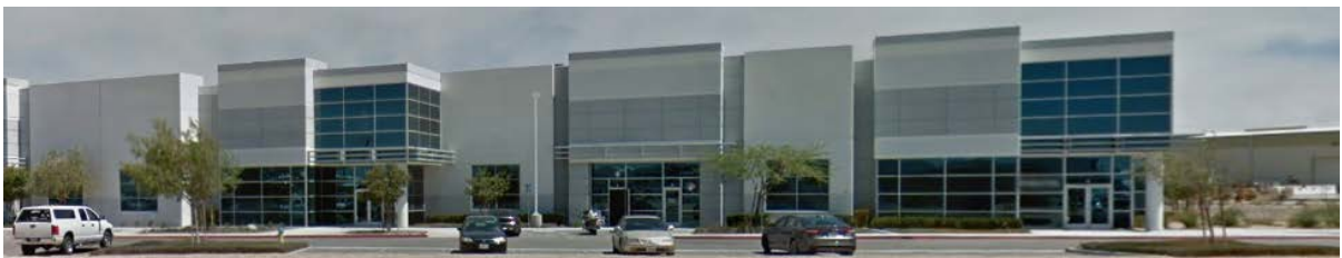
The entrance to Suite 2 is in the middle of this photo, with Suite 1A located behind the office to the right.
