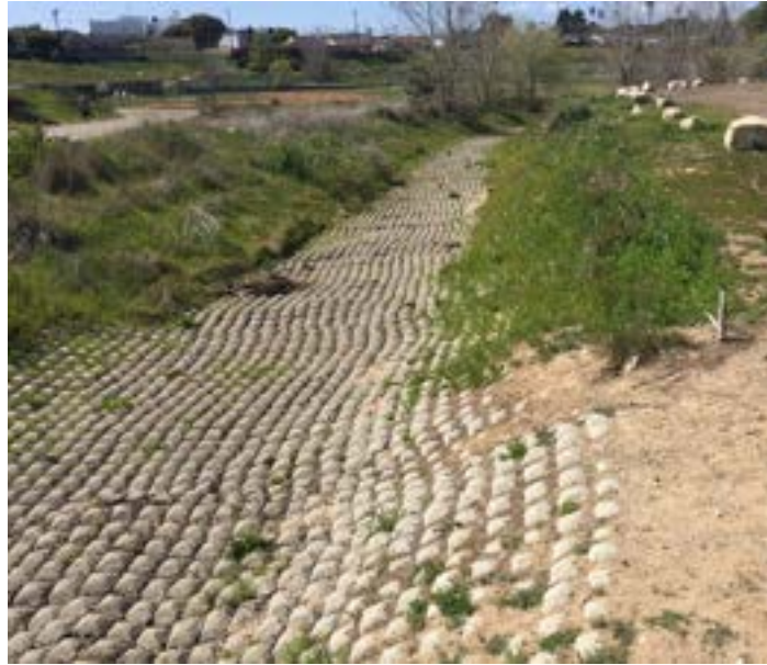
Figure 19: Vegetative Lined Channel with Reinforcing Mat
