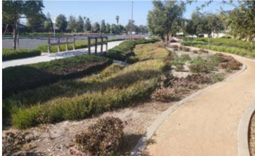
Figure 1: Example Linear Basin – City of Anaheim
