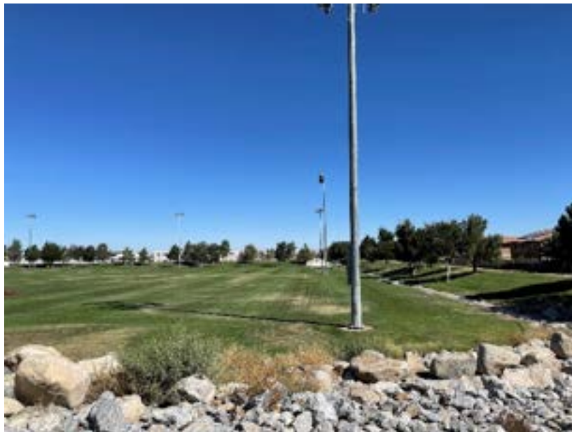
Figure 13: Multi-Use Detention Basin
