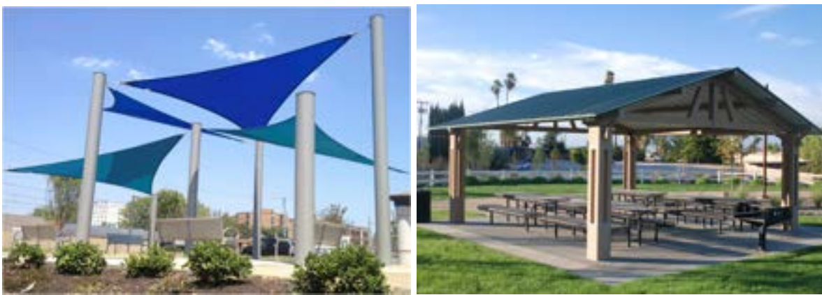
Figure 11: Shade Structures (Pictures by Poligon Shade Structures)
