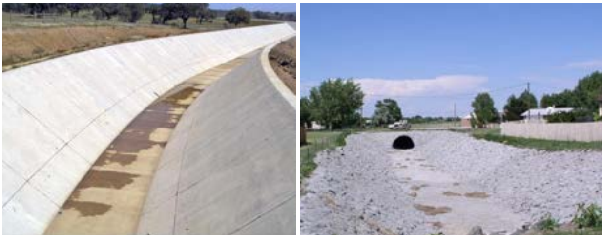
Figure 18: Hardscaped (Concrete and Riprap) Lined Channels
