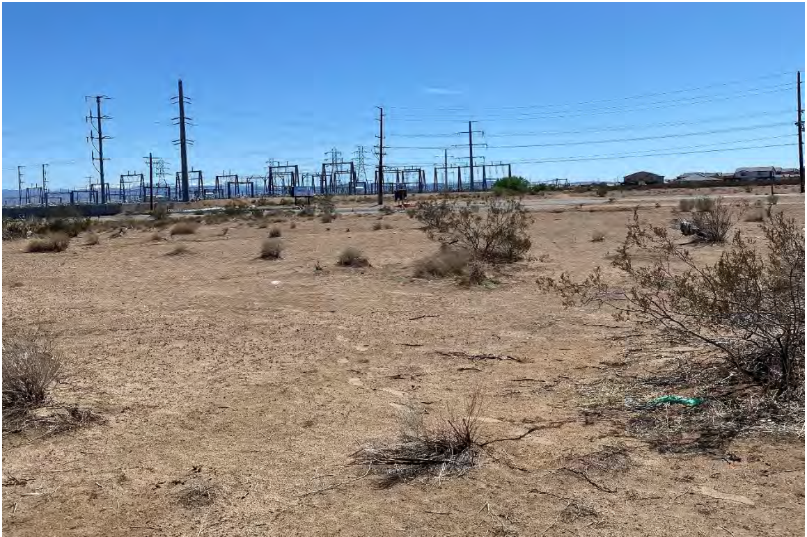
Photograph No. 3: Site, facing west.
