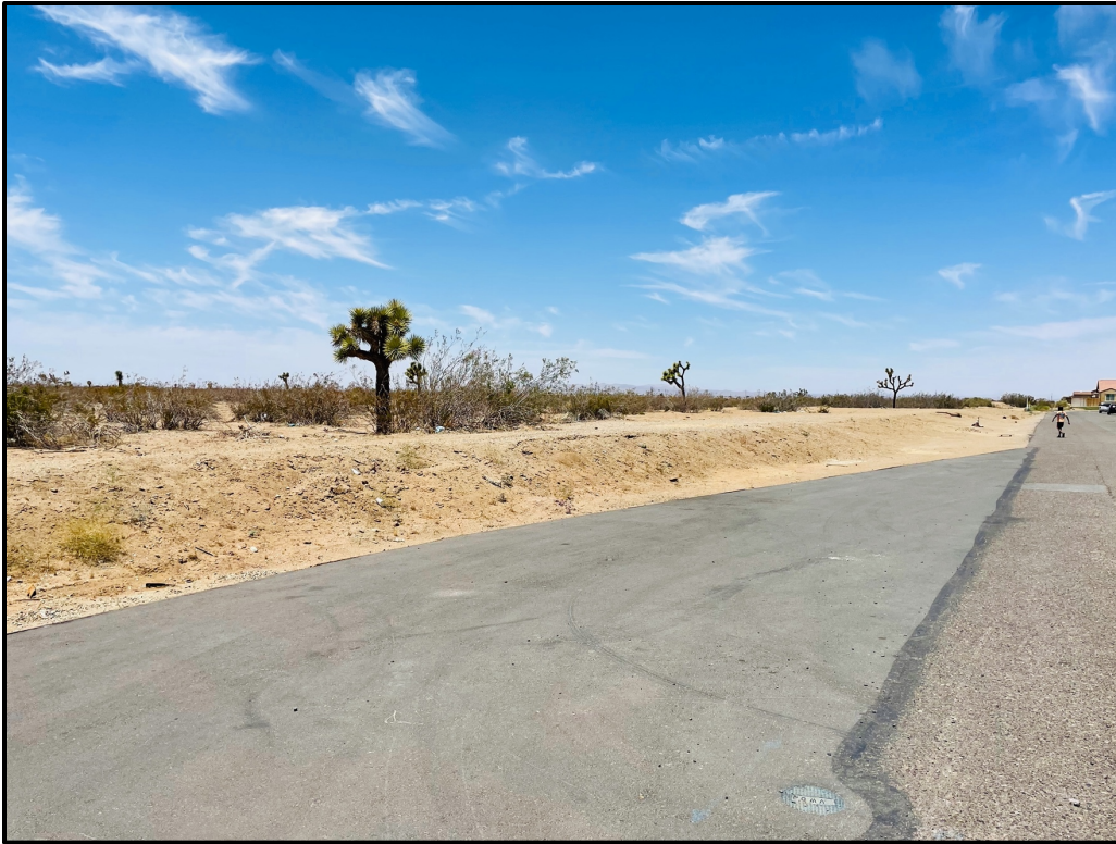
Plate 4.2–3: Overview of the project, facing north along Fremontia Road.
