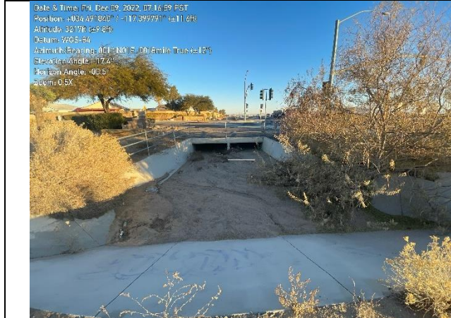
Box Culvert underneath Luna Rd. Facing North
