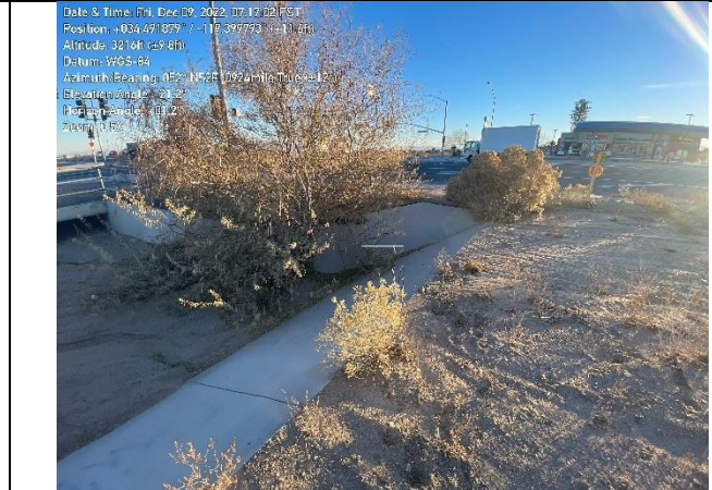
Box culvert at Luna Rd. and Hwy 395 Intersection
