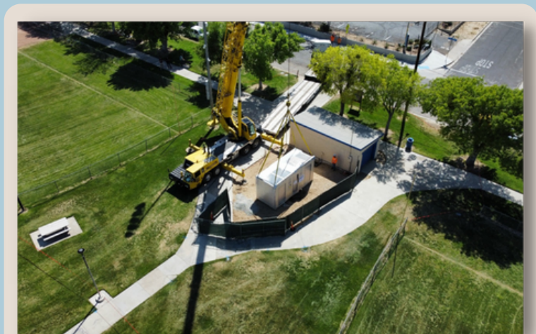
Installation of Brentwood Park Self Cleaning Restroom
