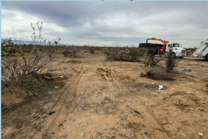
Public Works Encampment Cleanup
