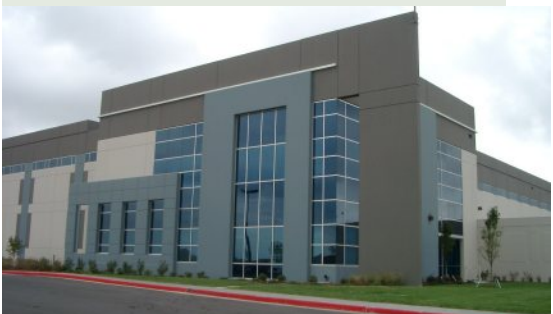
Figure 6.8 Light industrial building
