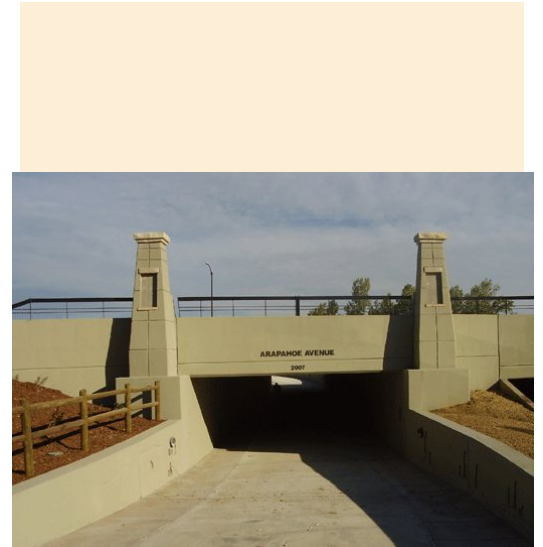
Figure 9.6 Dual trail and drainage culvert
