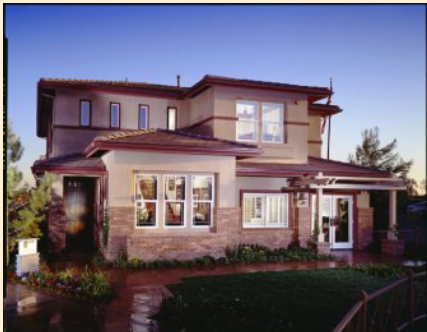
Fig 12.50 Contemporary example with entrance porch
