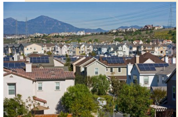
Figure 10.4: Housing with solar panels
