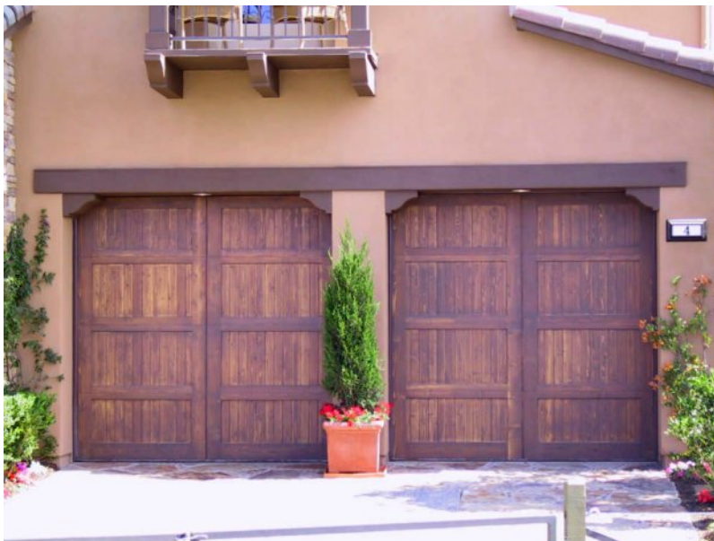
Fig 12.31 Garage doors that match the architectural style
