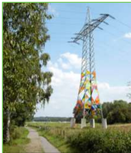
Students in Germany transform a transmission line tower into a “lighthouse” along a trail (Photo Credit: Julija Nèjè)
