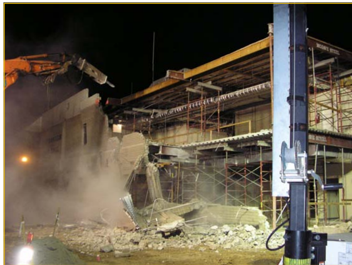
Demolition of a portion of City Hall
